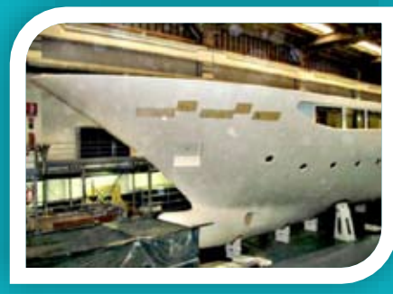
Installation sequence in Azimut-Benetti ship yard*
